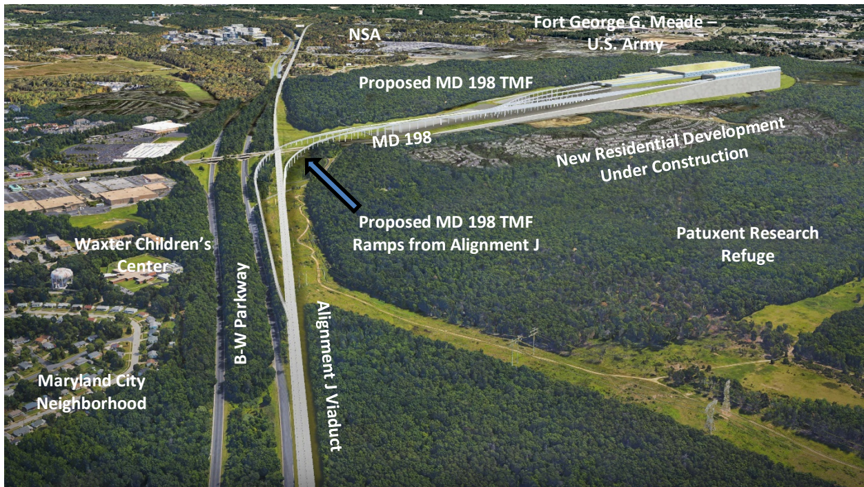
Figure 4.9-15: CAAs #10 and #12 - Illustrative Rendering of Proposed MD 198 TMF and Corresponding Ramps with Alignment J near Patuxent Research Refuge, Fort George G. Meade, and NSA, Looking North
