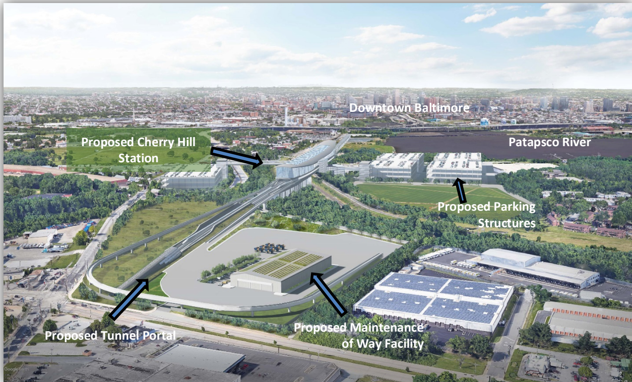
Figure 4.9-10: CAAs #18 and #19 - Illustrative Rendering of Proposed Cherry Hill Station, Tunnel Portal, Maintenance of Way Facility, and Parking Structures, Looking North
