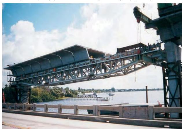
Figure 14. Balanced Cantilever Construction Method (Courtesy of WSP/Pace)
